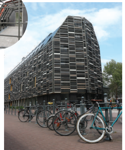
The Rizomm, situated at the core of the Université Catholique de Lille, at the heart of Lille, 41 rue du Port, designed by the architectural agency MAES.
